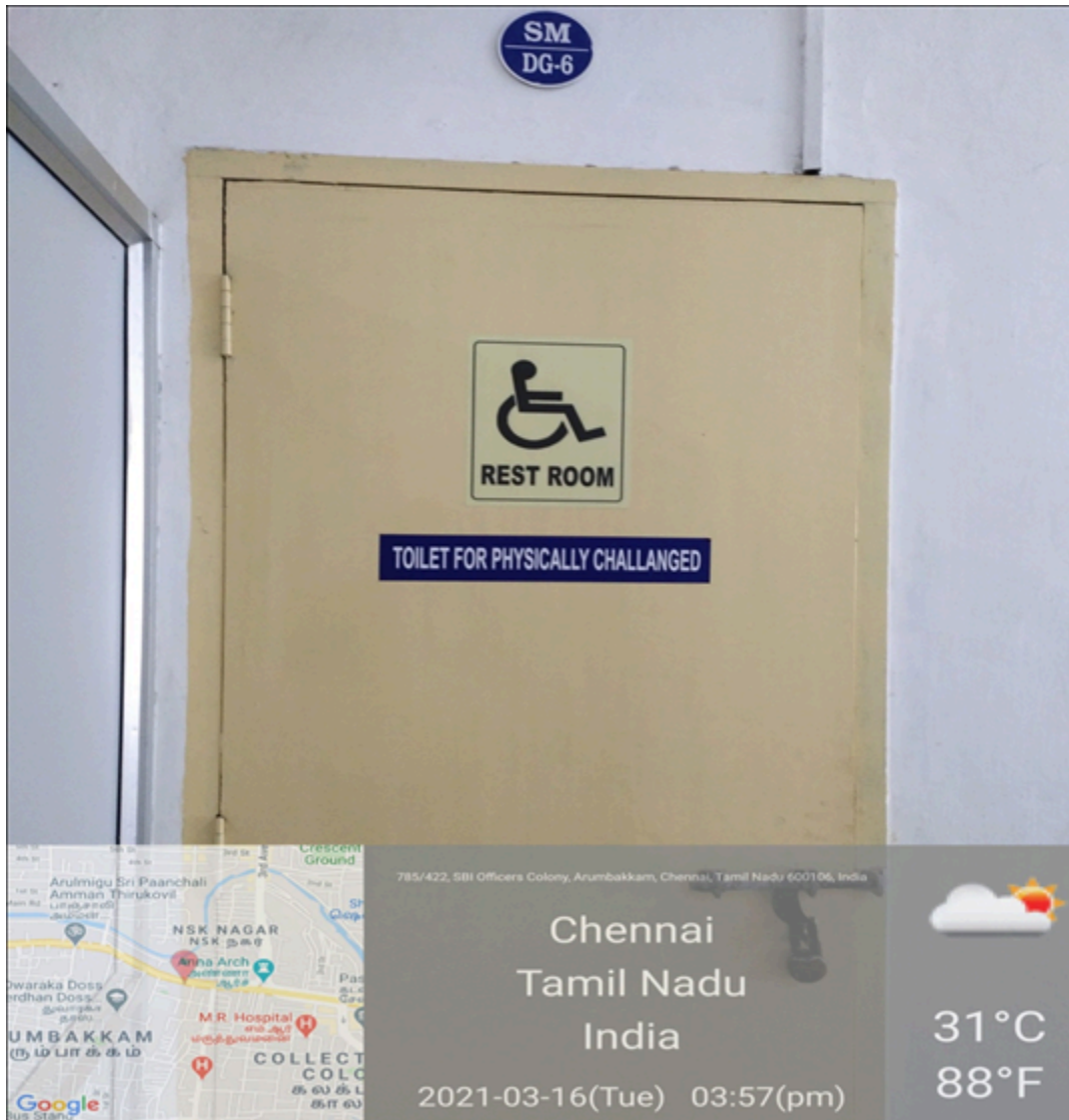
Disabled Friendly washrooms in MBA Block
