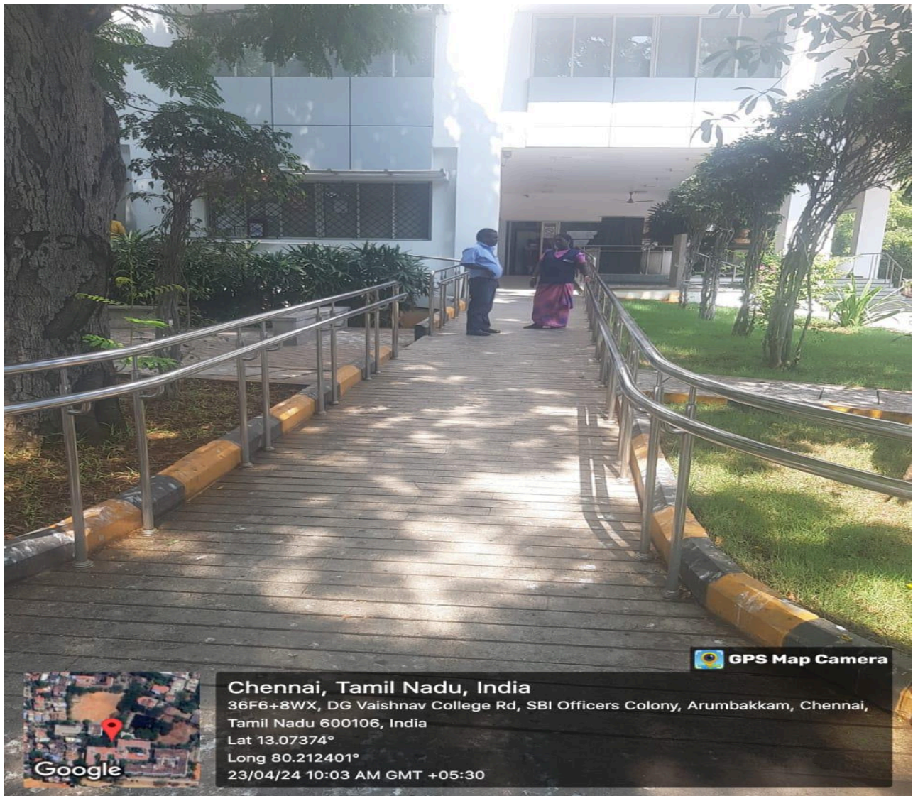
Ramp with Tactile Path near the Principal's Office
