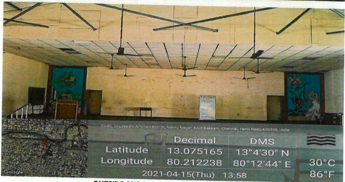
OUTSIDE AND INSIDE VIEW OF S. R.G HALL
